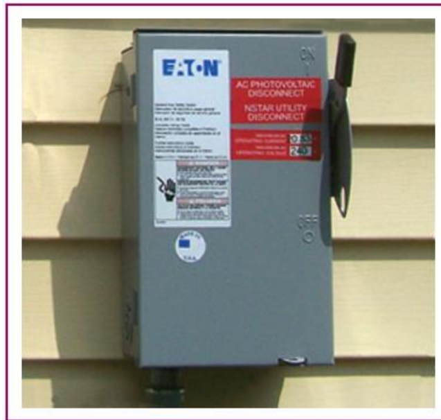
EXHIBIT 690.10 PV system disconnect.
